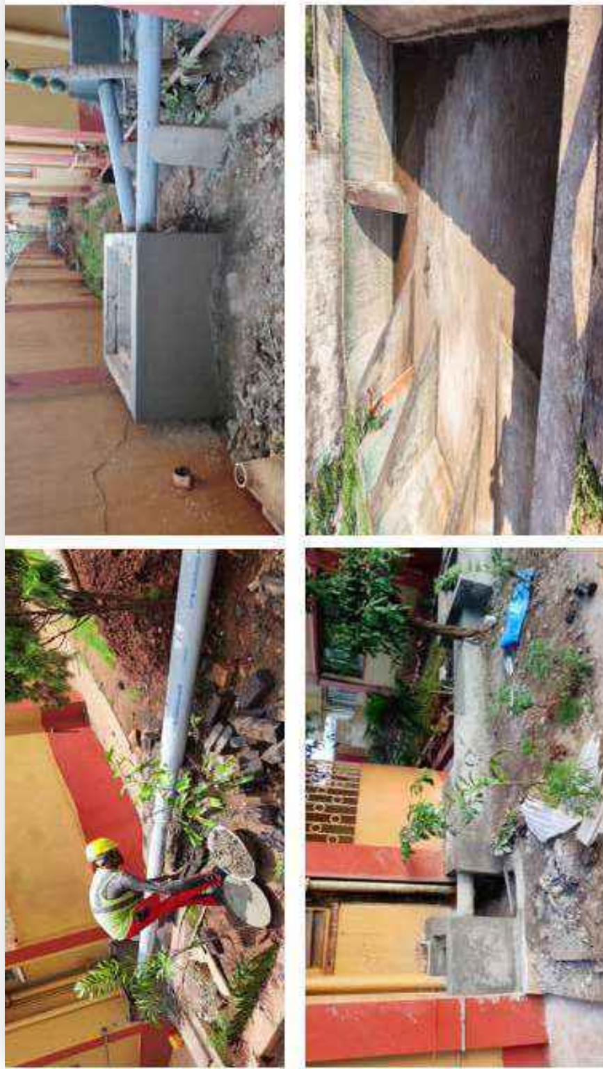
Rooftop Rain water harvesting system
